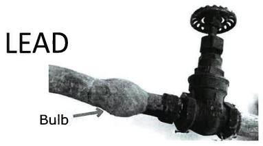
A dull, silver colored pipe that can be easily scratched with a coin or key. Scratching leaves a shiny silver color. Magnets <u>WILL NOT</u> stick to lead pipes. Lead pipes are bendable and commonly have a "bulb".
